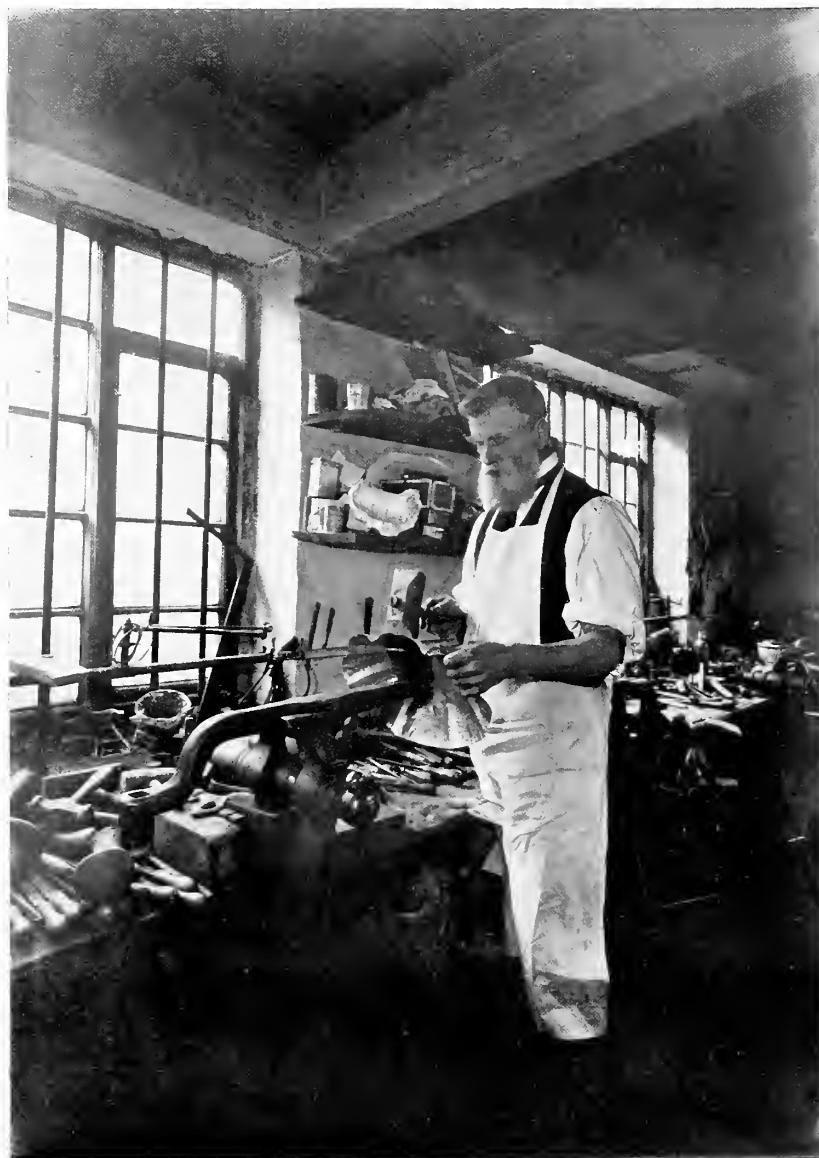
2 — Illustration of Raising by hand.
