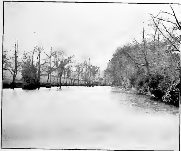
Dam from which power was derived.
