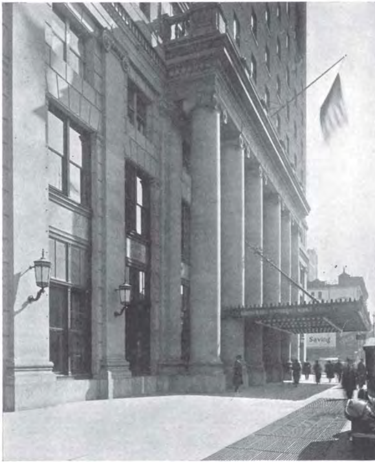
Detail of Main Entrance on Seventh Avenue
