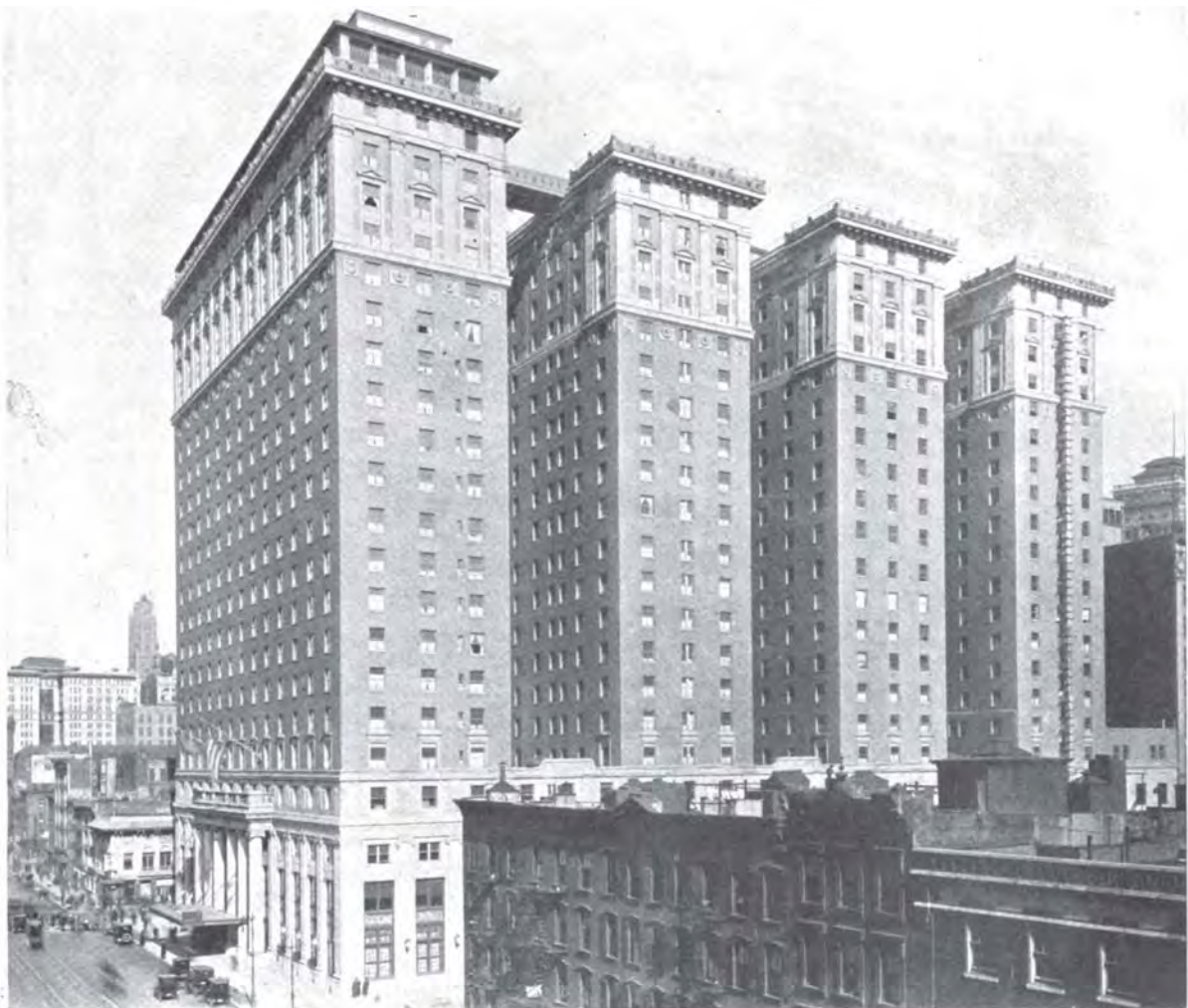
General View of Hotel Pennsylvania from Southwest
