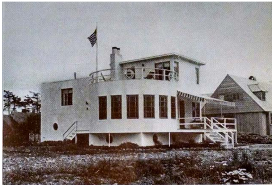
"Complete house, inside and out, is constructed of Resnprest Durez bonded plywood. Note the smooth rounded surfaces"
